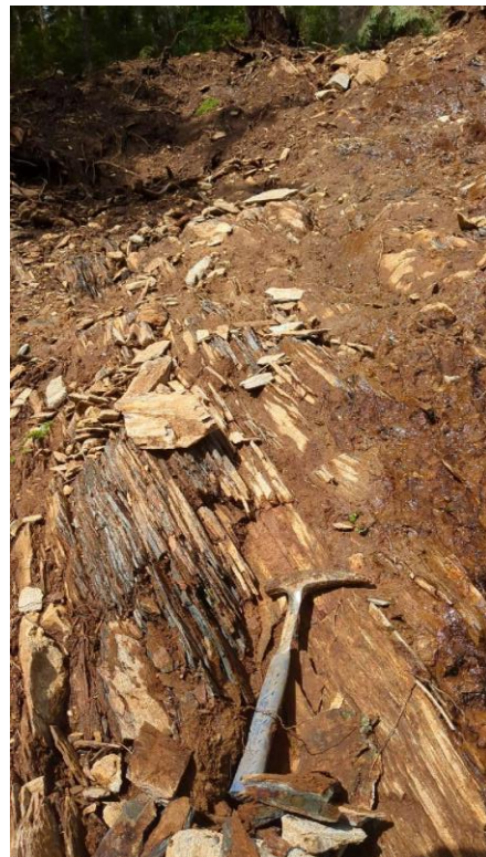
B: Copper Ridge Landslide, Point 1037, Upper Zone, phyllite bedrock exposure.
