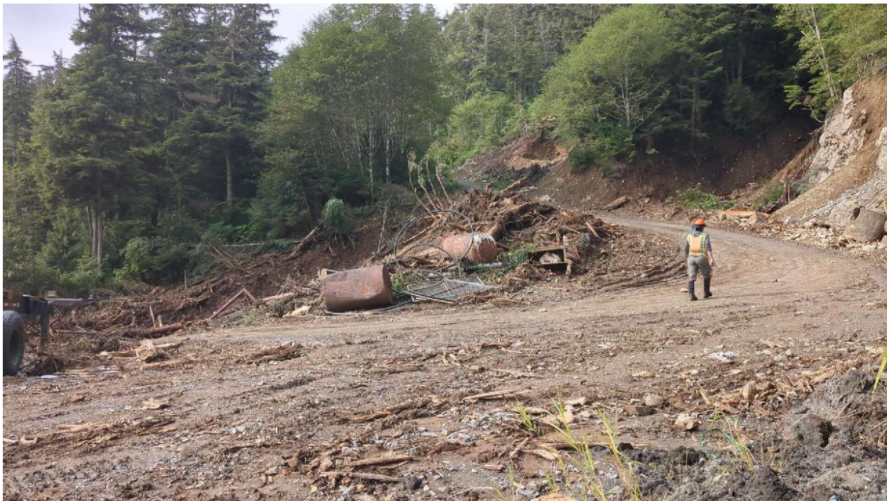
B: Copper Ridge Landslide, Point 1022, Lower Zone, debris accumulation at access driveway switchback.
