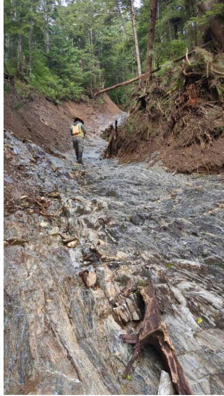
A: Copper Ridge Landslide, Point 1023, Middle Zone conditions with scoured bedrock exposures.
