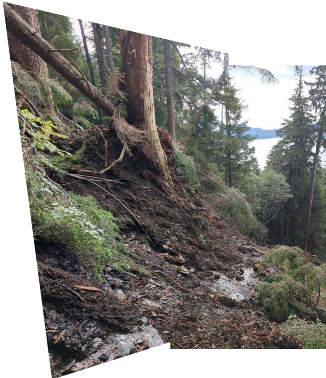
B: 3rd Avenue Landslide, Point 30, colluvium deposits under an isolated tree within slide mass.
