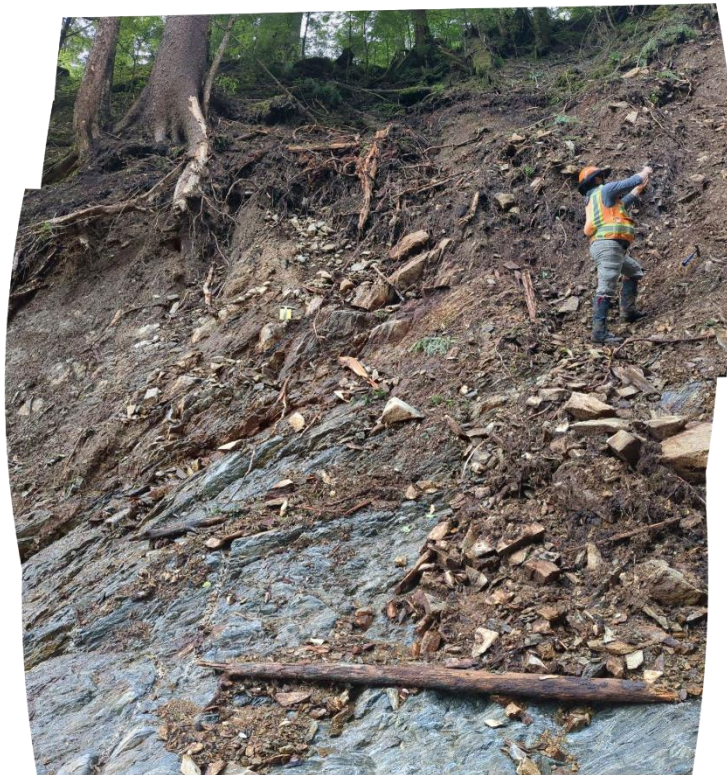
B: Copper Ridge Landslide, Point 1024, Middle Zone conditions with colluvium exposures.
