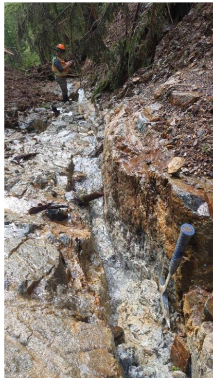
B: Copper Ridge Landslide, Point 1059, Middle Zone fault gouge in upper scoured stream channel looking southeast.
