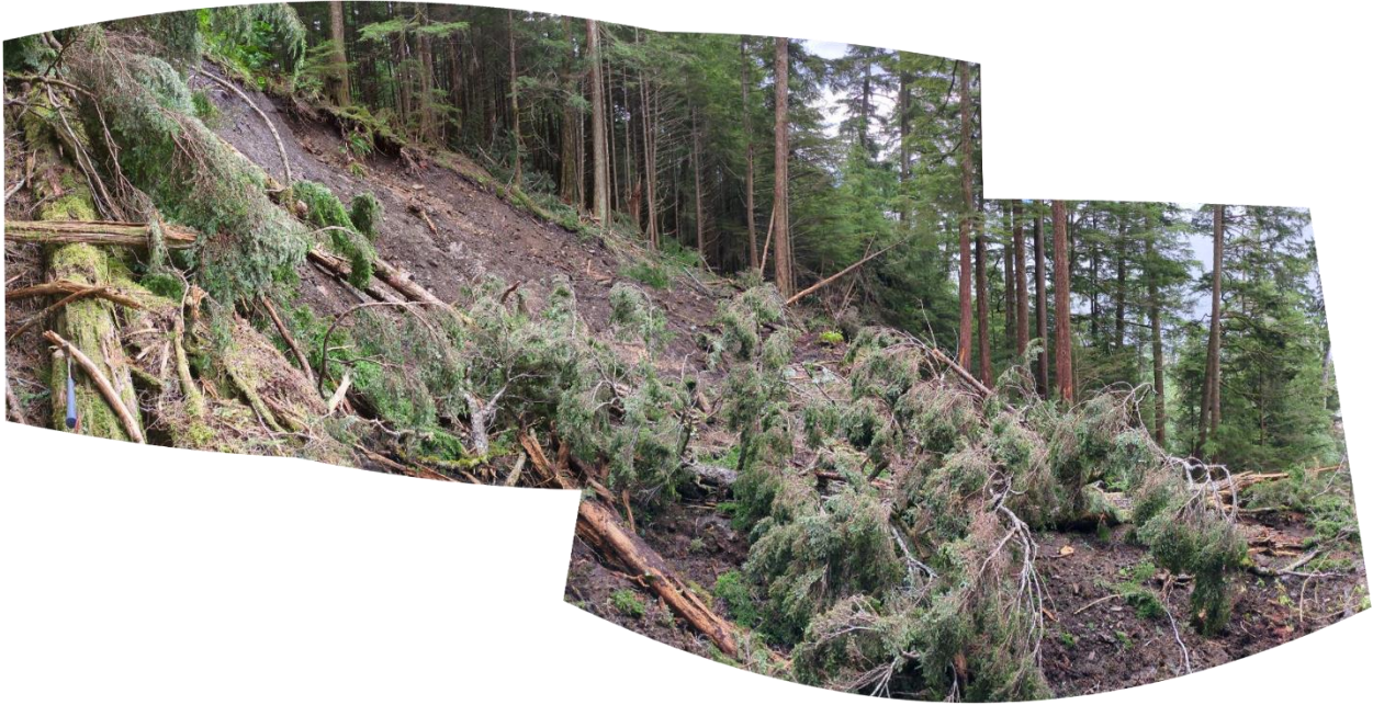
A: 3rd Avenue Landslide, Point 37, colluvium deposits.
