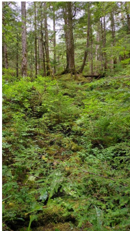
B: 3rd Avenue Landslide, Point 43, wet area upslope of landslide headscarp.
