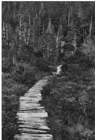
Trail development through much of the Central Gravina landscape will require boardwalks and other surface treatments to permit year-round use.
