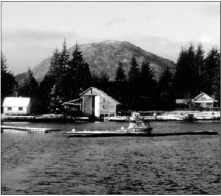
This boat maintenance structure on the Stensland property in Clam Cove is the community's most prominent landmark. It was first constructed in the early 1900s. Note that the building next to it is on skids and was brought in by water; often the easiest way to get a house in an area without roads.
