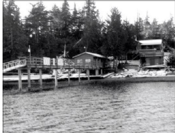
Development on shoreline lots without road access requires investments in some kind of mooring or docking structure. Where nearshore topography is shallow, such as in this case along Tongass Narrows south of Clam Cove, a lengthy dock may be necessary. Where more intense shoreline development happens, such structures could be shared by both waterfront and upland property owners to reduce construction and maintenance expenses, minimize environmental impacts and reduce clutter along the shoreline.
