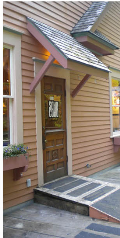
Shed Roof Marquee Creek Street
