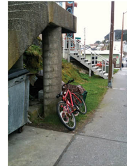
The Inman St. stairs provide the only street-side area for the residents above. Parked bicycles, garbage receptacles, and other items spill out onto the sidewalk. This area may be organized to better meet neighbor needs and landscaped with street trees and flowers to be more attractive.
