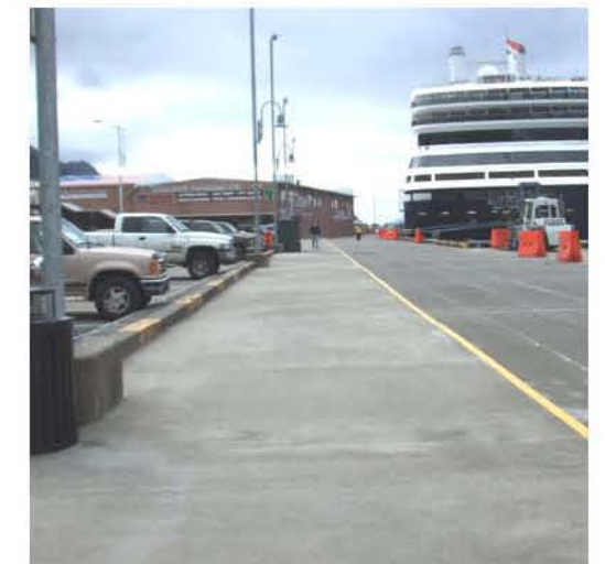
Existing Site-Berth 3 looking south
