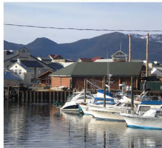
EXISTING SITE FACING EAST
