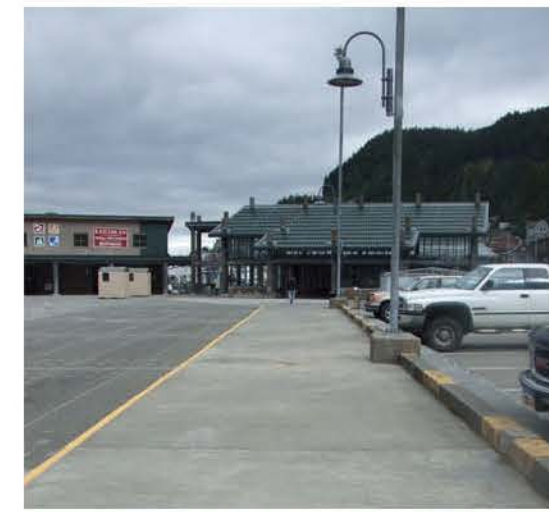
Existing Site-Berth 3 looking north
