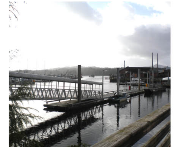
5. Existing Thomas Basin Float 6
