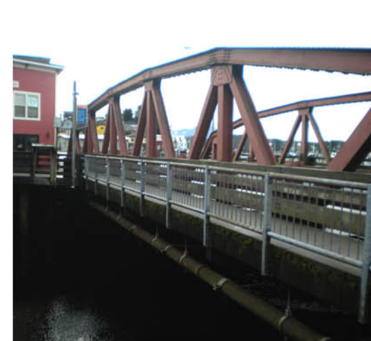
4. Creek Street Bridge Sidewalk
