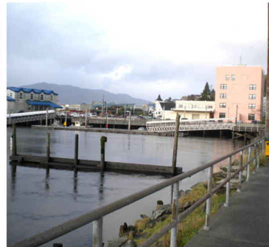
3. Existing Stedman Street Breakwater
